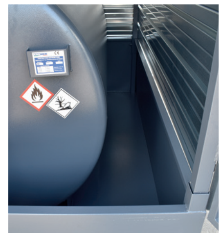
Accessible interior for cleaning and maintenance
