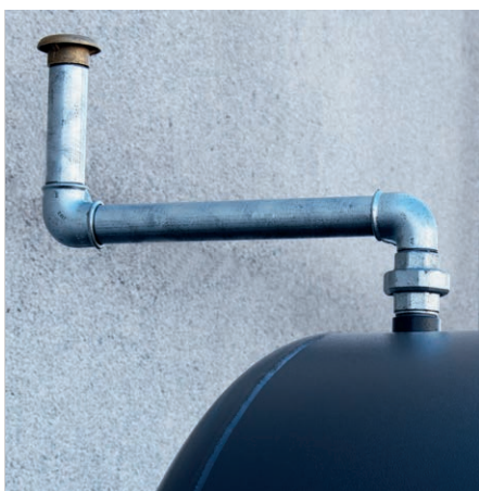
Pressure relief valve with flame-breaker mesh
