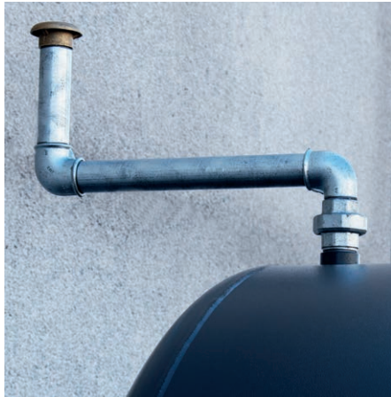
Pressure relief valve with flame-breaker mesh
